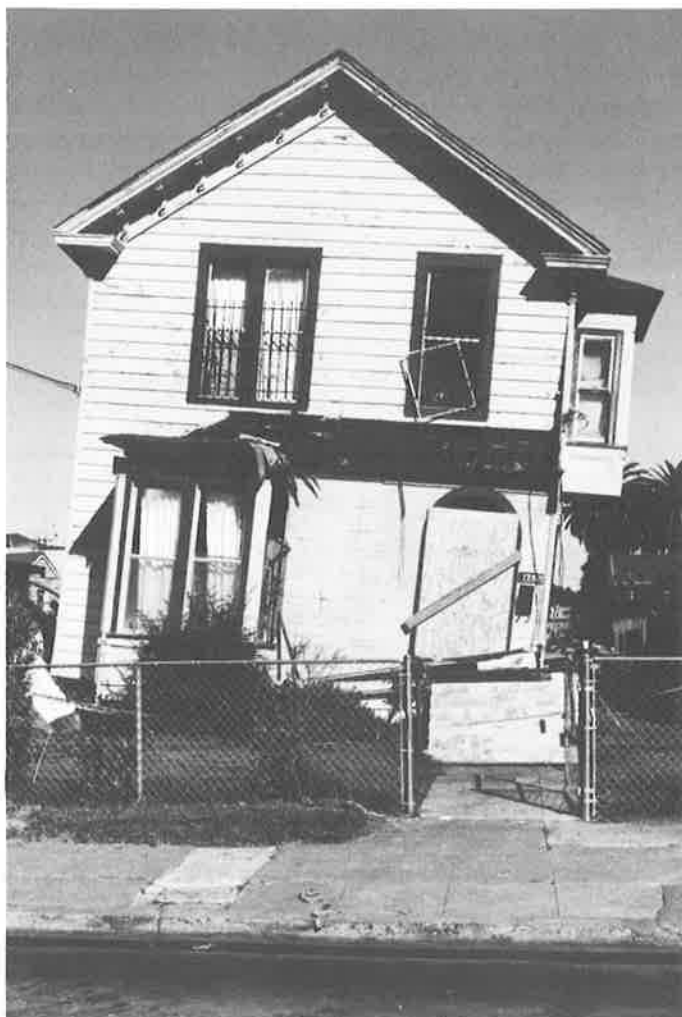
1416 11th Street, 1871-72, in the Oakland Point district: one of several West Oakland Victorians demolished. Below, the Shorey House, 1782 8th Street, was one of the lucky ones: it came off its foundation but is now being repaired. Captain William Shorey, who lived here from the 1880s to the 1910s, was a whaling master; the Shoreys were leaders in the Bay Area black community. (Muffy Kibbey/OPAT)
