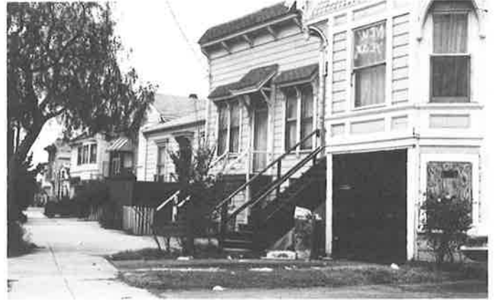
West Oakland survey is uncovering the history of a vast area of intact 19th century working people's housing, like this block of Peralta Street. You can help. (Phil Bellman)
