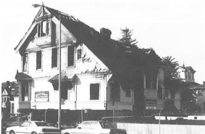
Herrick House before (Pill Hill, 1985) and after: latest landmark to perish by fire. (Phil Bellman)
