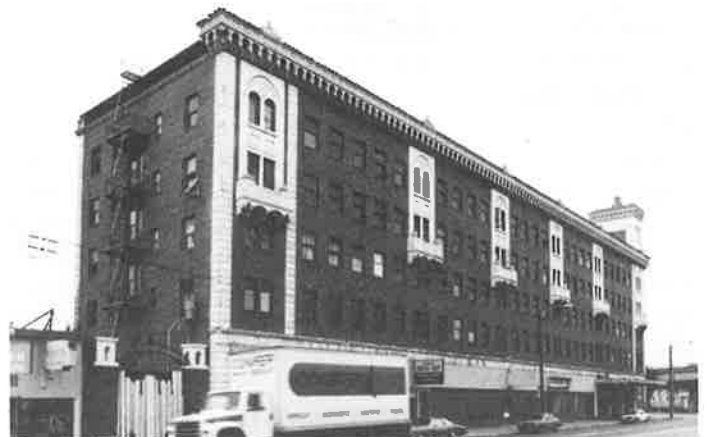
California Hotel (Clay Burrell, architect, 1929), placed on the National Register. Oakland Community Housing Inc. is rehabilitating it as low-income housing. (Survey photo)
