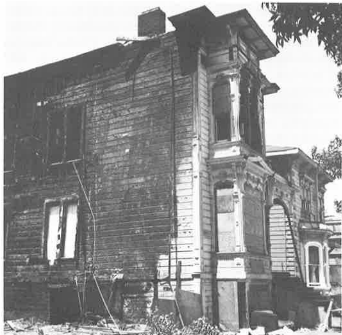
Wetmore houses on 11th Street downtown--burned amid controversy over landmarking, demolition, and housing; and
