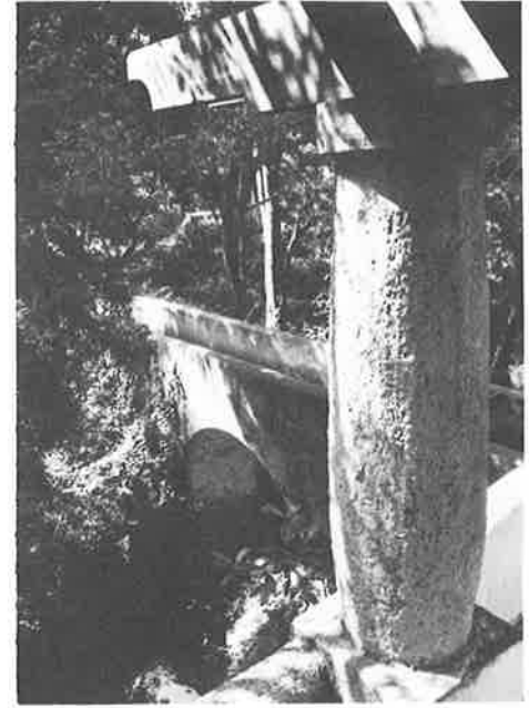
Creek, bridge, and pergola with tile-trimmed columns. (photos, Phil Bellman)
