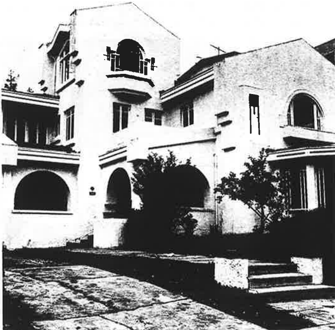
Locke House on Harrison Street (John Hudson Thomas, 1911) is a magnificent example of Viennese Secessionist style. Owners are making use of incentive which allows commercial uses in landmark houses in certain zones. (Phil Bellman)
