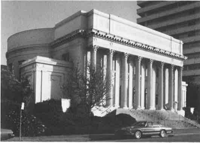
Former Fourth Church of Christ, Scientist, 1330 Lakeshore Avenue: demolition controversy began in June 1986, may be coming to a close. (Randolph Langenbach)
