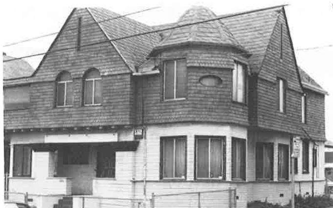
Another converted residence, 836 36th Street housed the Black YMCA in the late '30s. (Phil Bellman)
