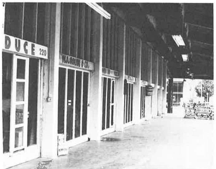
Early morning bustle turns to midday ghost town. Screened fronts, high transoms, bold signs, and corrugated metal canopies make the market buildings unique. (Gary Knecht; Oakland Cultural Heritage Survey)
