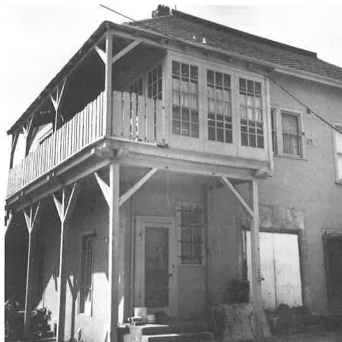
Charlie Tepper's hotel building survives behind stores at 2030 MacArthur Blvd. (Phil Bellman)
