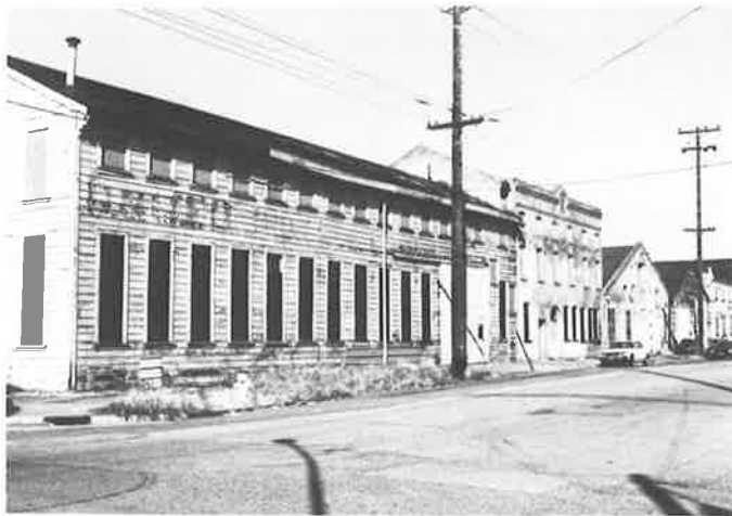
Oakland Ironworks: frame building in foreground has been retained and refurbished (1982 Survey photo)
