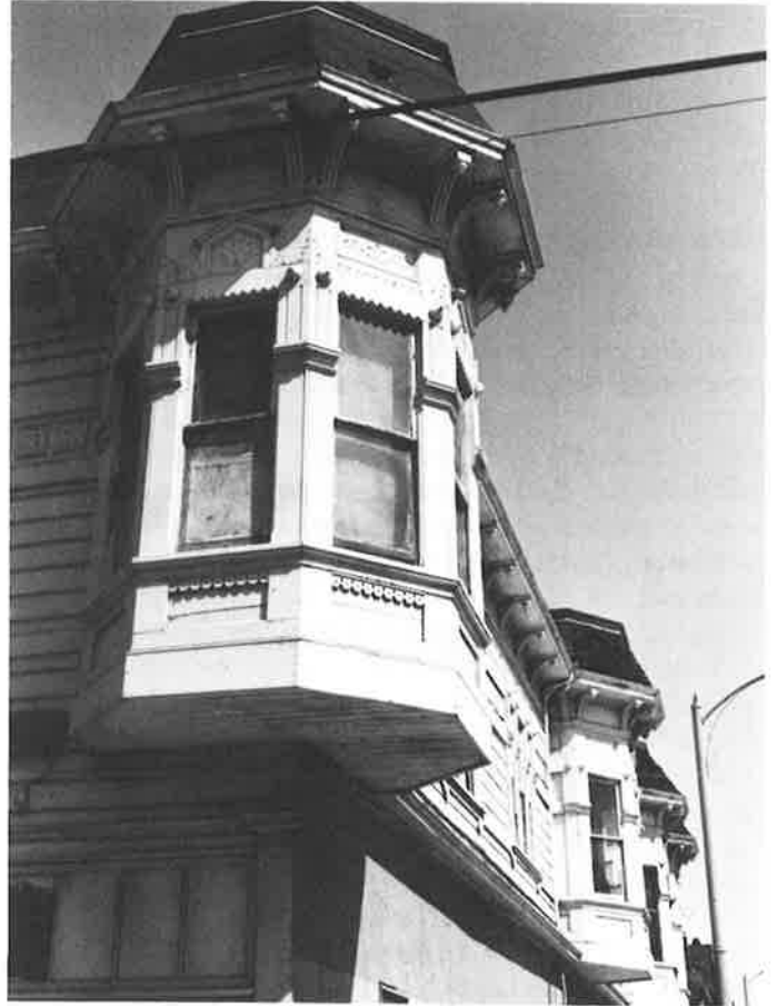
Central Building, 1101 East 12th Street: Italianate landmark demolished by the City (Survey photo)
