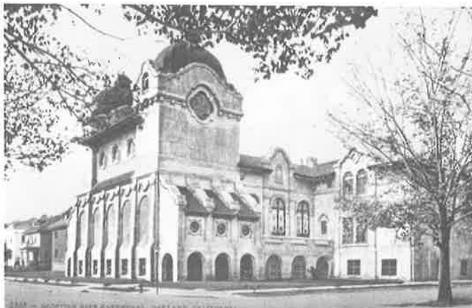
Mission Revival style Madison Street Temple: one of the buildings for which Survey's and Board's ratings differ. (1910s postcard)
