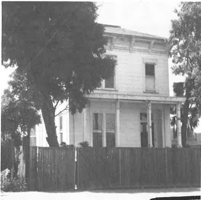
The original Fannie Wall Home (1918-28), at 1215 Peralta Street.
