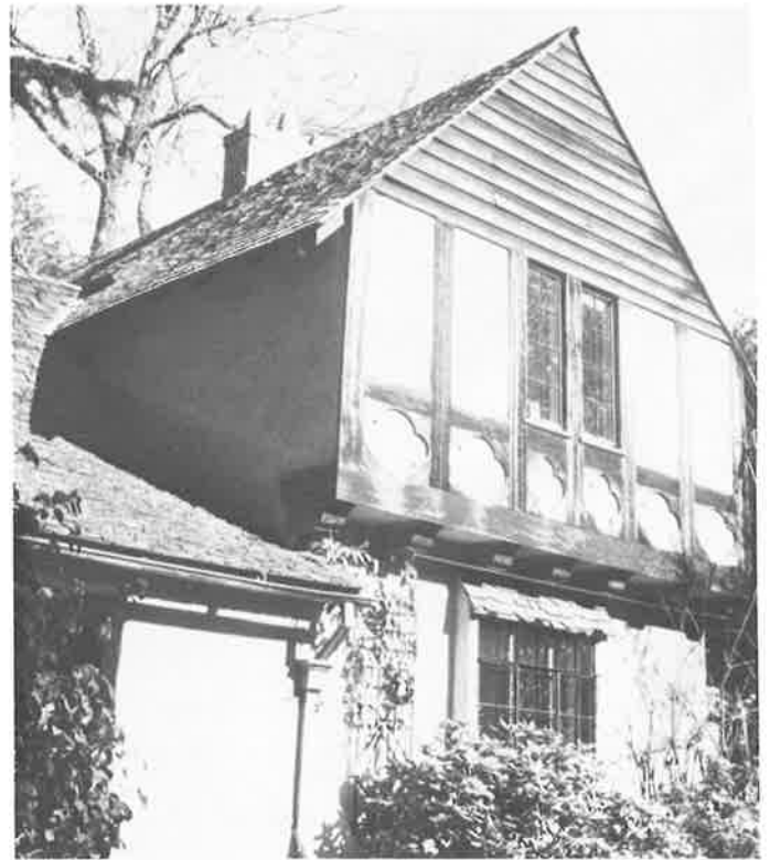
1508 Fernwood: another variation on the English cottage, designed in 1928 for Alvah Judson Rogers by an unknown architect. (photo by Edward Phillips)
