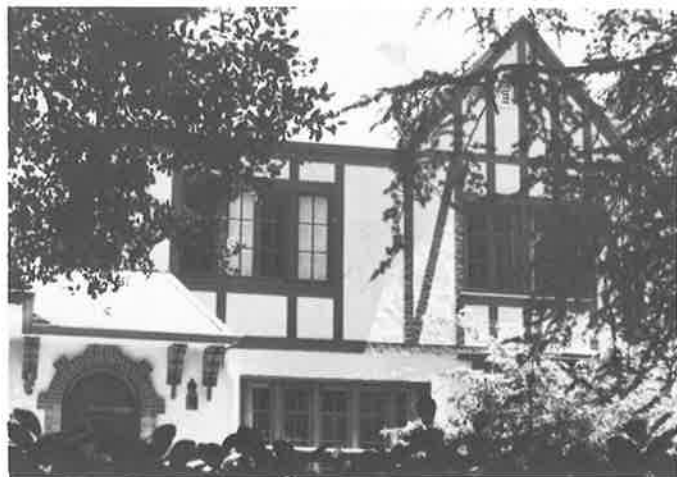
Half-timbering is one of the characteristic period costumes for Fernwood houses. (Edward Phillips)
