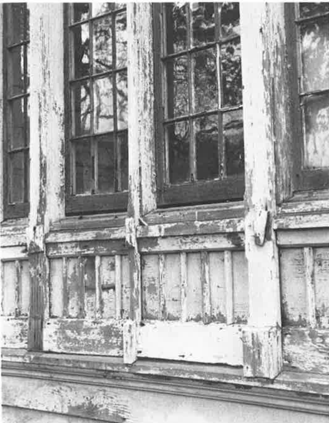
Anatomy of a Stick villa: Cohen house (above and R) urgently needs paint and repair. (Phil Bellman)
