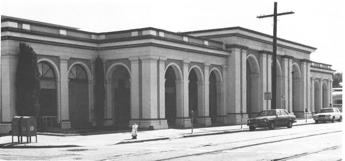
A stop-work order was issued after alterations to the exterior of the first building designated a city landmark were begun without review by the Landmarks Board.
