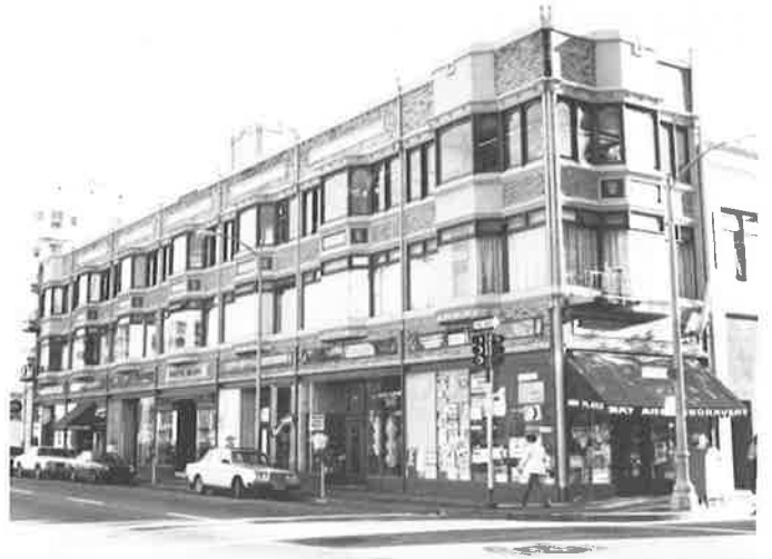
The White Building at 15th and Webster (Clay Burrell, 1924-25), new city landmark (Survey photo)
