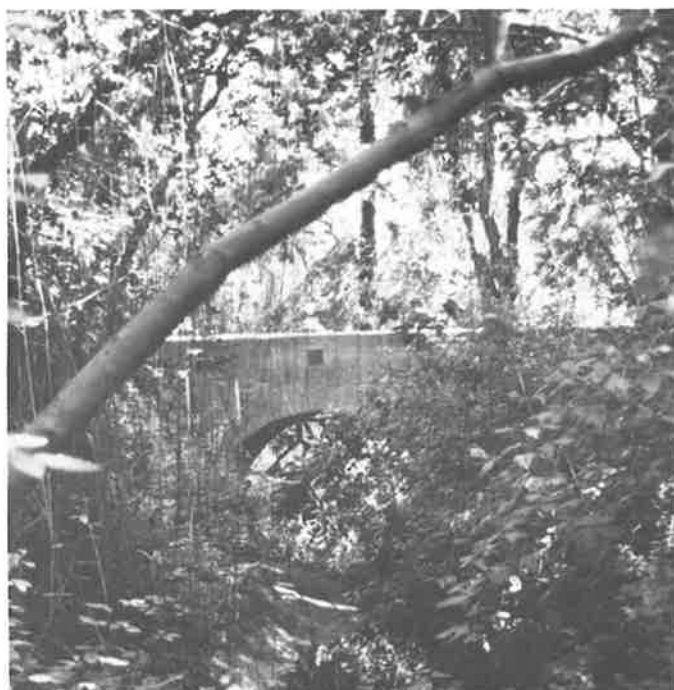
Glen Echo Creek: bridge in Oak Glen Park, designed by Oscar Prager in 1910 (Survey photo)
