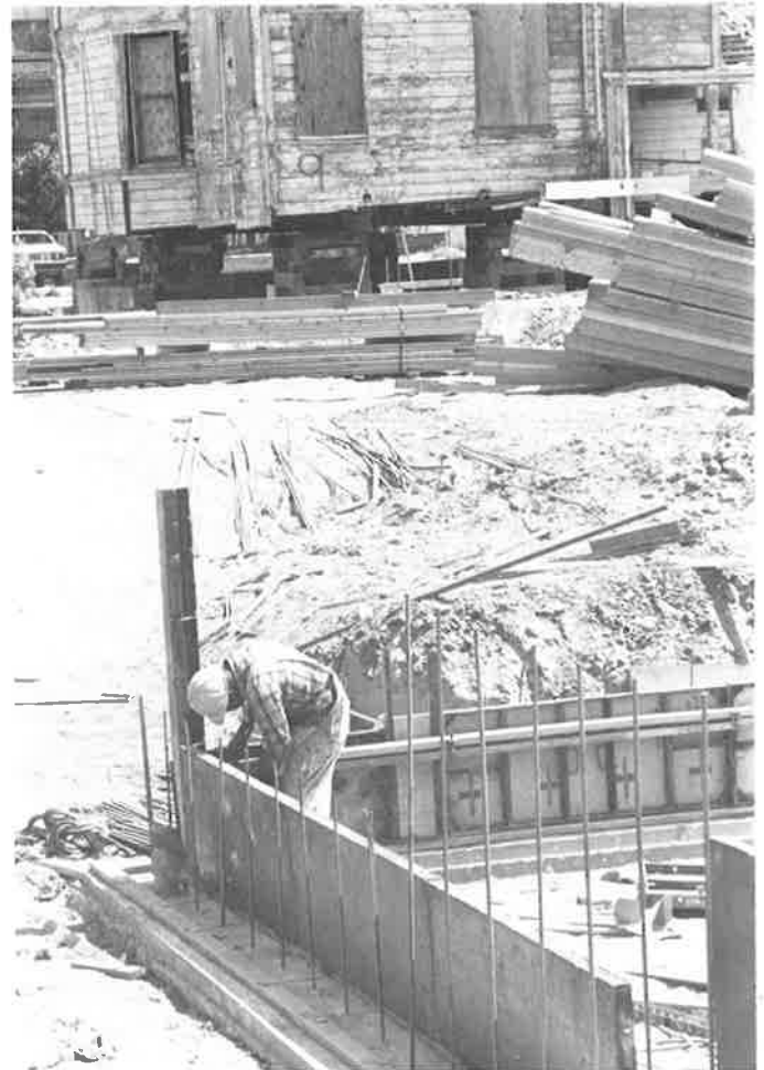
work in progress at Preservation Park (Phil Bellman)
