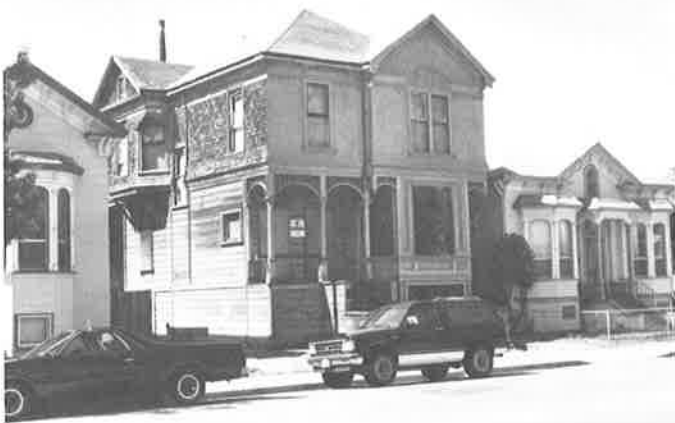
The Hoover House, 1079 12th Street: endangered, but not endangered enough (photo: Phil Bellman)
