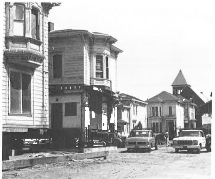
Work proceeds at Preservation Park (Phil Bellman)
