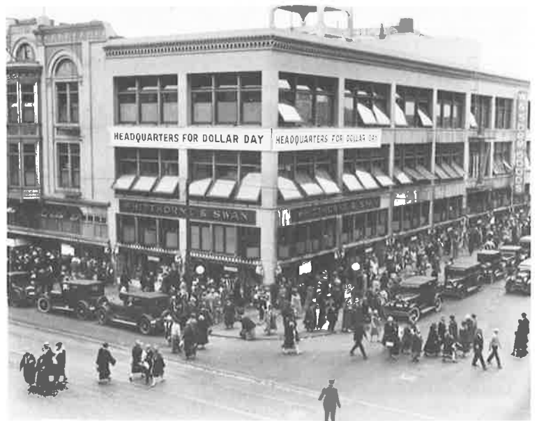
Whitthorne and Swan, c. 1928 (Photo: Oakland History Room)
