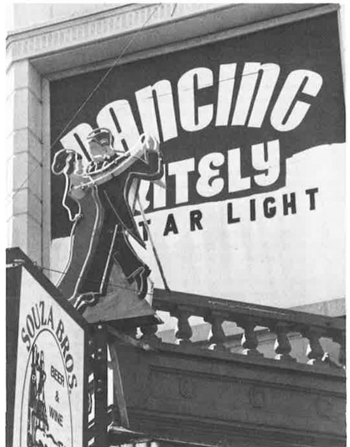
The Starlight Ballroom (Weber Block) at 12th and Webster, is slated for demolition if the Hotel II project becomes a reality.
