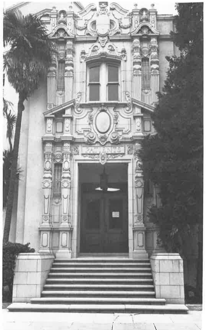
A terra-cotta inscription marks the patients entry into the corridors of the administration building, elaborate enough to dispel any stigma attached to going to a public hospital.
