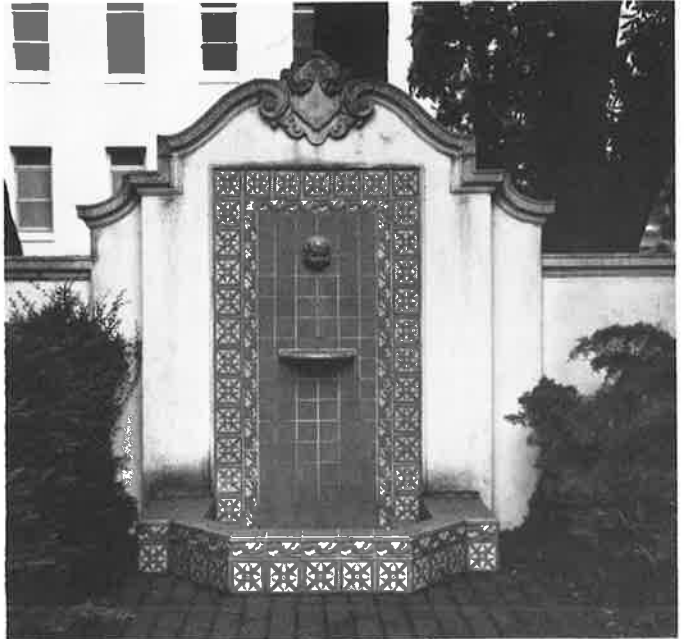
Detail of a fountain in one of the courtyards flanking the administration building, part of the park-like grounds designed to encourage patients' speedy recovery.
