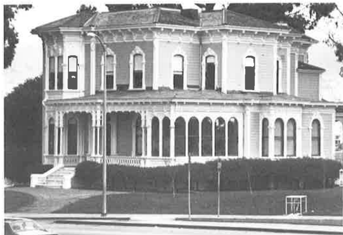
Camron-Stanford House will receive $148,000 towards its continued restoration.
