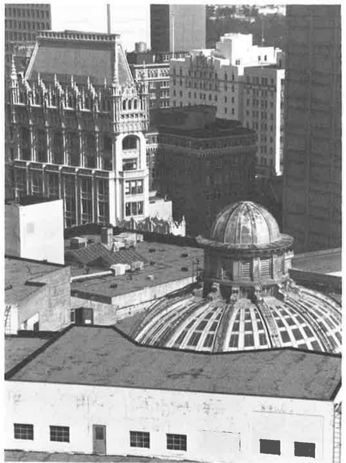
The unique oval glass dome topping the Liberty House Building towers above Broadway across from the Cathedral Building.
