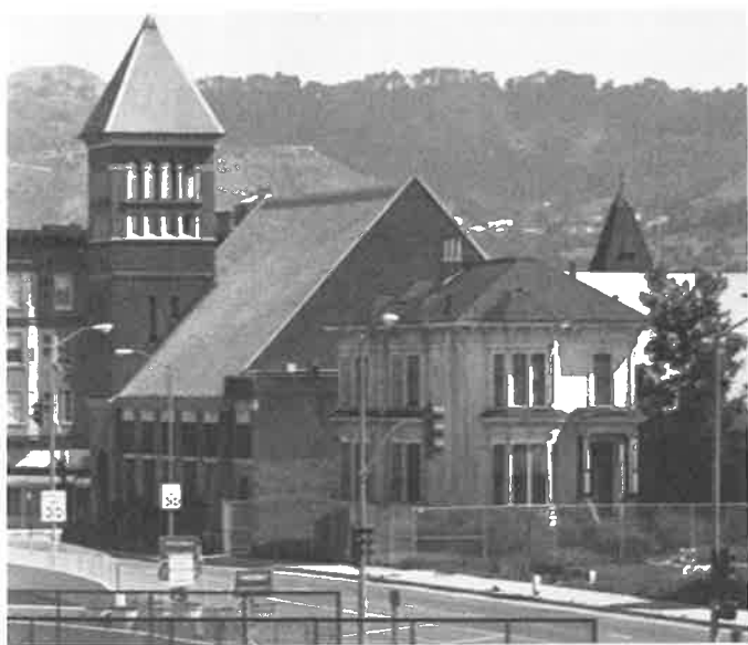
The First Unitarian Church, adjacent to the Highway 24 downtown extension, was one of three Oakland landmarks to receive preservation grants. It is a cornerstone in the planned Preservation Park project.
