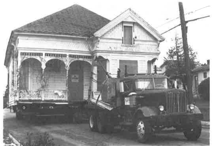
On Sunday October 30th, this Queen Anne house was moved from its original location on Dimond Ave. to a new home in Preservation Park where there are now 12 structures awaiting rehabilitation.
