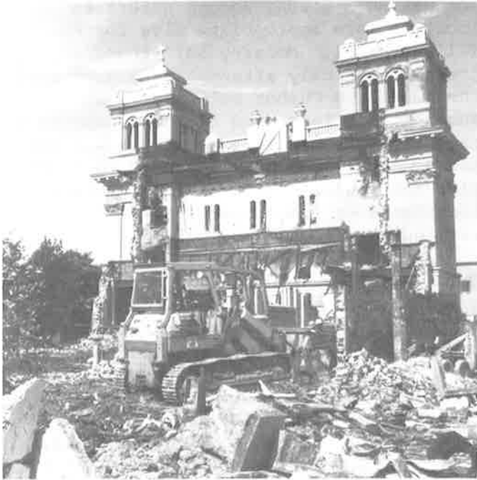
Gone and lost forever. The fire-damaged shell of the once magnificent First Methodist Church was recently reduced to rubble.
