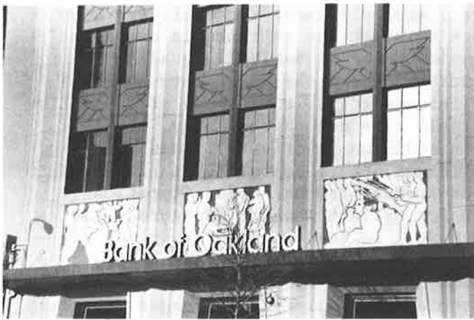
Bank of Oakland Building, 360 14th St., John Stoll & F. Reimers, 1928. The stylized eagles and the s'graffito panels were acclaimed for their "modern" inspiration.
