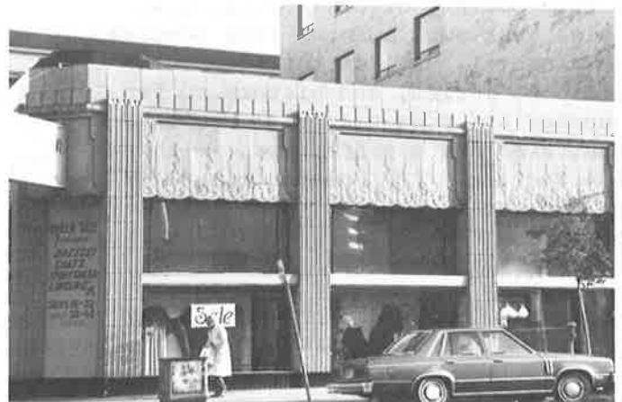
Roselyn Dress Shop Building, 14th & Harrison Sts., C.W. McCall, 1931. The terra cotta is pale green. The panels above the windows appear almost as curtains raised on the fashion show inside.
