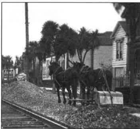
OAK CENTER TRACK RECONSTRUCTION: In 1918, the tracks on West 16th Street, looking east from Chestnut Street (right), were given fresh new sidewalks—you can see the “before and after” on either side of the tracks. The photo above (from a nearby street) shows how horses graded the material.
