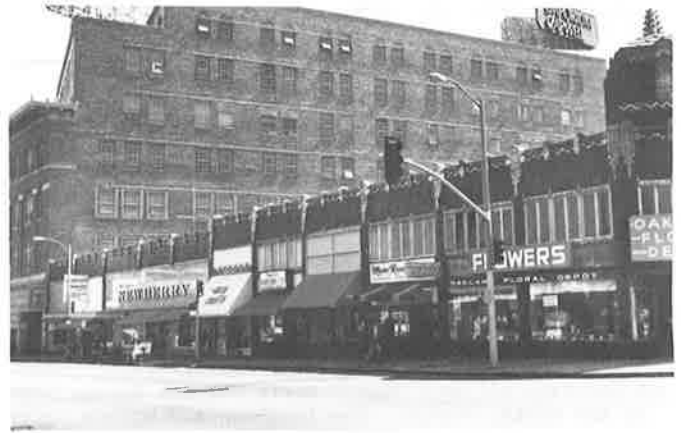
Floral Depot and Newberry Building, next to Emporium-Capwell (Telegraph Avenue side)
