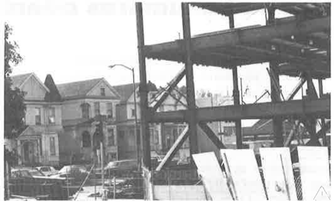
ABAG/MTC Building under construction at Madison Square, facing Victorian homes
