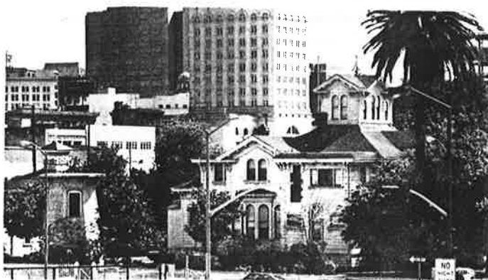
The Pardee Mansion (1868) in Preservation Park, with Oakland City Hall (1914) in the distance
