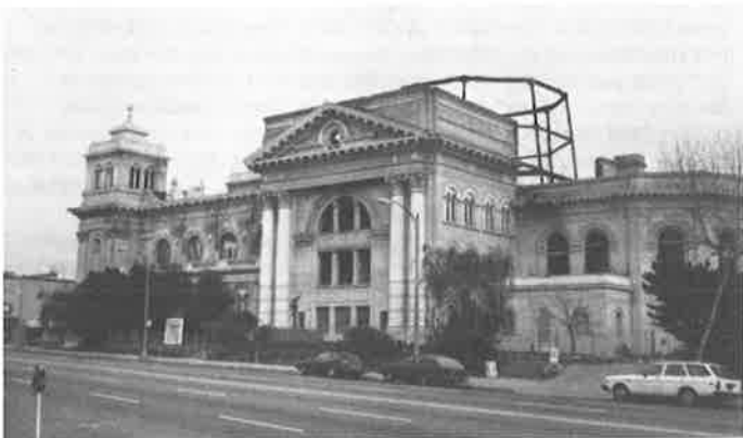
Fire-gutted shell of First United Methodist Church, 24th Street and Broadway
