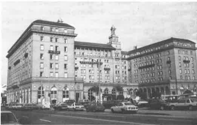
The Hotel Oakland, recently rehabilitated as senior citizens' apartments, will be one case study illustrating the theme, "Reinvesting in America," at the preservation conference April 29-May 2.
