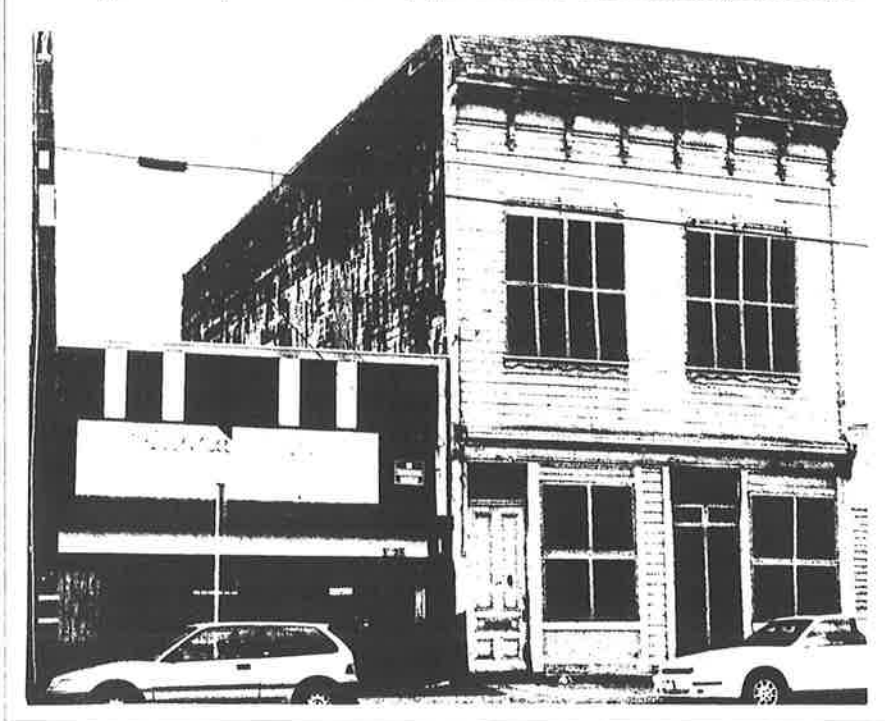
The vacant Fruitvale Hotel doesn't look like a boarded-up eyesore -- the windows have been simply but cleverly covered with black paper to resemble intact windows. (Jeanette Sayre)
