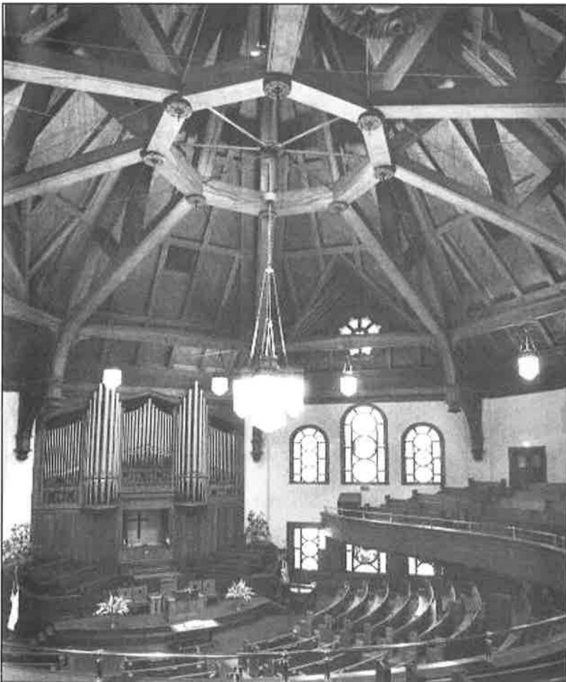
The First Baptist Church auditorium designed by Julia Morgan in 1906 features an open-timbered roof made of redwood. ( Sara Holmes Boutelle )
