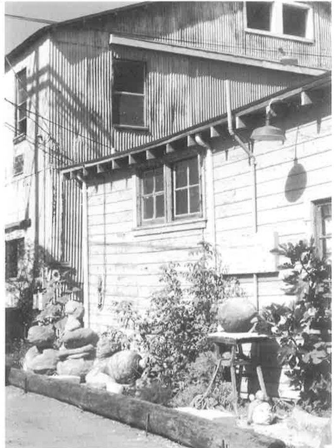
More to life than money: utilitarian Hurley Marine Works buildings now foster ceramics, painting, poetry, and invention. (Robin Bartoo)
