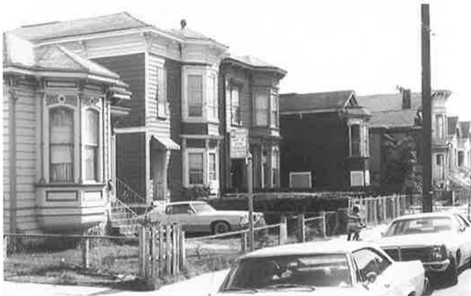
Oakland Point district, isolated for 35 years by the Cypress Freeway, is a prime example of Stanley Lowe's statement that "often people have gold in their neighborhoods and don't recognize it." The Italianate and Queen Anne at right have been on Code Compliance's demolition list. (Survey)
