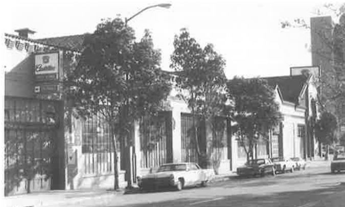
Harrison Street frontage of Cox Cadillac: Rite Aid's "preservation alternative" proposed to remove the service wing and keep this wall as a freestanding screen or trellis: City is requiring an EIR. (Survey)
