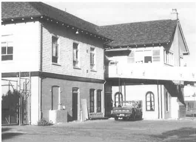
Studio One building, originally the Ladies' Relief Society Children's Home, faced the middle of the block toward the Society's other homes, for infants and elderly women. Roof shape dates from 1906 fire repairs. (Survey)
