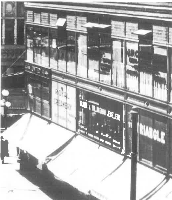
Board is concerned about appropriate period signs and awnings on the unusual high glass base of the Plaza Building next to City Hall. (Survey)
