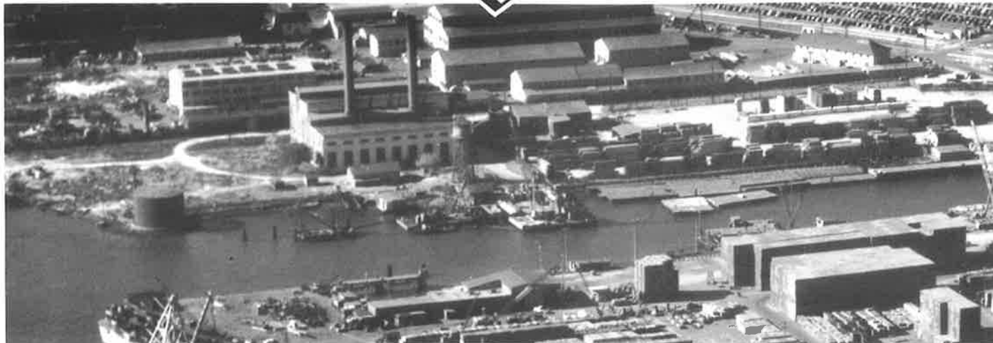
Another Sunderland aerial from the mid 1940s: Hurley Marine Works from the southeast. Building with smokestacks in front and right of the Plate Shop is the Great Western power station. Across Clinton Basin in the foreground is the open cargo area of the 9th Avenue Terminal (City Planning)
