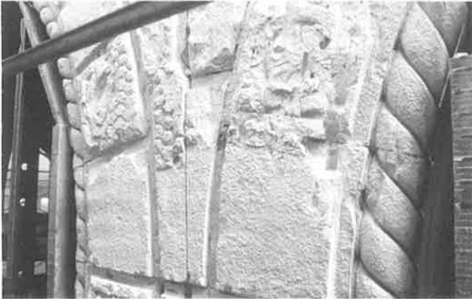
Central Building's 1925 terra cotta arches, as well as parts of the ornate bank interior, emerged during remodeling. Could they be reused or restored? Only the next generation may find out. (Chris Candell/CEDA)
