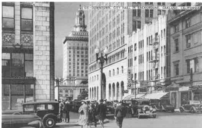
View up 14th Street from Franklin is little changed today: left to right, Financial Center Building, City Hall, Central Building, Elks Club, and Athenian-Nile Club (now Geoffrey's). (postcard c.1940)
