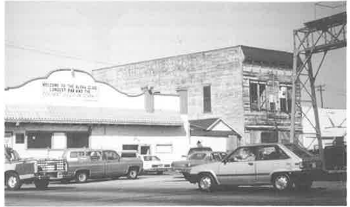
Fruitvale Hotel & friends: trackside location flanked by saloon and signal bridge illustrates "integrity of setting, feeling, and association." (Survey)
