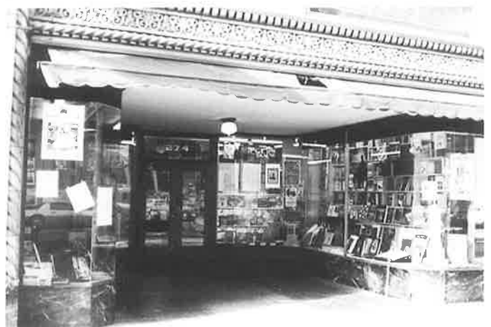
Holmes storefront: even improved Demolition Ordinance and Preservation Element won't prevent work without permits. (Survey photo, 1982)
