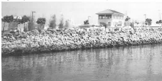
In 1874 the Army Corps of Engineers created the modern Oakland Estuary by dredging and constructing stone Training Walls on the Oakland and Alameda shores. Port proposes to replace Oakland's north wall with additional container berths. (Betty Marvin)
