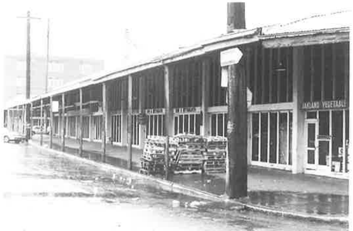
Unique special-purpose 1916 buildings in the Produce Market figure in both the Estuary Plan and the Magnificent Seven (p.8). District designation could recognize their importance and guide future use. (Survey)
