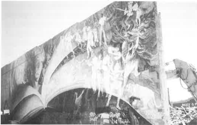
The 1925 Gilson Electric building (rated "C") was demolished this summer at 11th and Madison, and with it this 1988 mural, "An invitation to read, and to understand," by Brooke Fancher and Kriska Boiral. (Betty Marvin)
