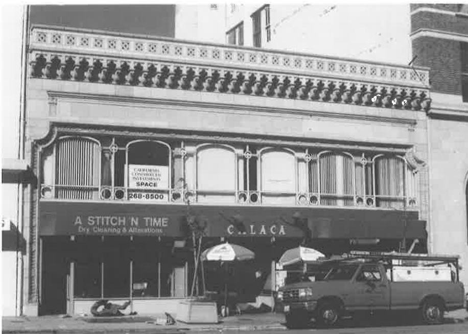
1611-19 Clay Street today. The neighboring PG&E building also had a notable sign: see page 17.
