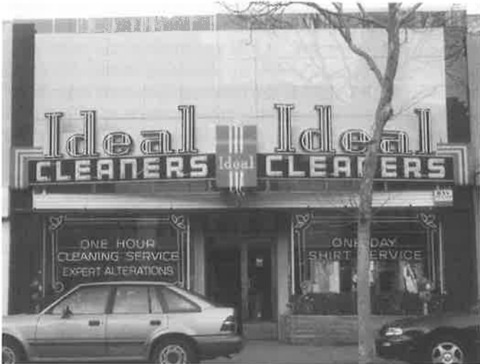
Ideal Cleaners, 322 14th Street: The multicolored neon complements the multiple colors of the Vitrolux glass facade. The clean line and rounded form of the canopy indicate a 1940s date. (Michael Crowe; Betty Marvin)
