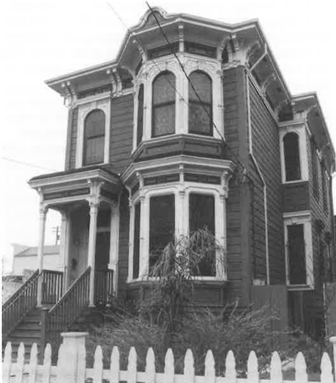
This house on 8th Street, eligible for the National Register as a contributor to the Oakland Point District, was restored by Jubilee West. (Bill Coburn)
