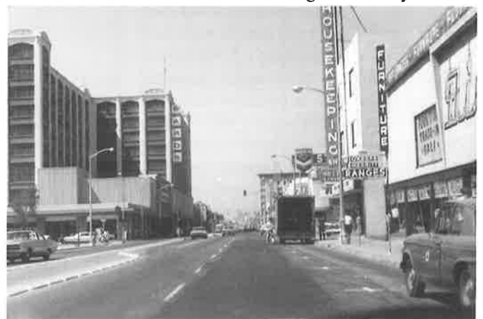
This 1967 City Planning photo shows the Ward's building as the largest of a cluster of furniture and department stores in the "second downtown" in Fruitvale. (Oakland Cultural Heritage Survey collection)
