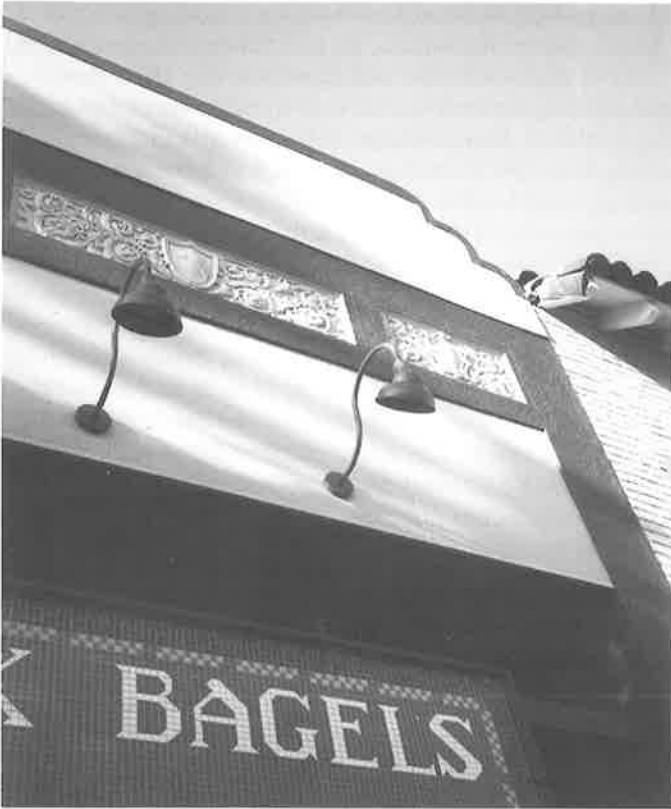
A long-hidden frieze is revealed on the former Toyhouse building on Lakeshore. Scallops on the parapet recall the shape of the mid-century metal cladding. (Carolyn Douthat)
