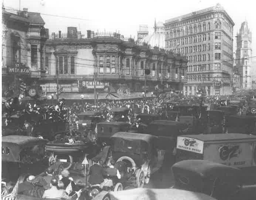
Armistice Day 1918, looking north from 13th and Broadway. Three monuments of Mayor Mott's time - the Rotunda, Broadway, and Cathedral Buildings - rising above their Victorian neighbors, as well as the throng of motor vehicles, give a sense of the rapid modernization in Oakland in the Progressive era. (Oakland History Room)
