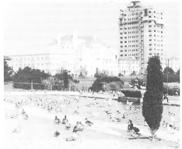
This view across the lake in 1929 shows the Bellevue-Staten under construction, the Women's Athletic Club, and several other buildings in the Bellevue-Staten Apartment District proposed for S-7 designation.
