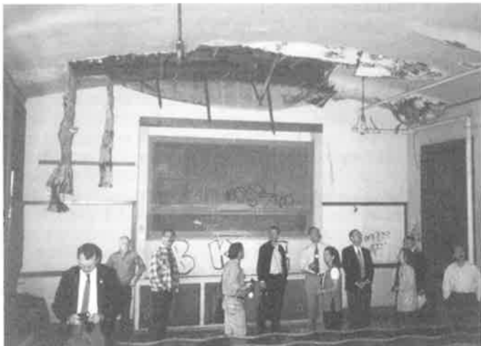
National Park Service representatives recently toured Old Merritt. Historic interiors like the lecture hall (with metal lath hanging from the ceiling) still appear threatened by intent to offer tenants "white boxes," minus blackboards and moldings. (NOVA)
