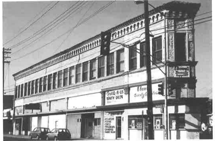
This ornate flatiron marks the "hub" of East Oakland. Is that the world's smallest building at far left? Come on Andrew Carpentier's new Foothill-Seminary walking tour this summer and find out. (Survey photo)
