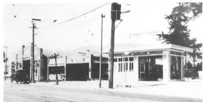
Union Oil erected the steel station shown here (its second gas station on the site) in 1920. The brick garage at left was demolished when Safeway expanded. (Berkeley Historical Society, Louis Stein collection)
