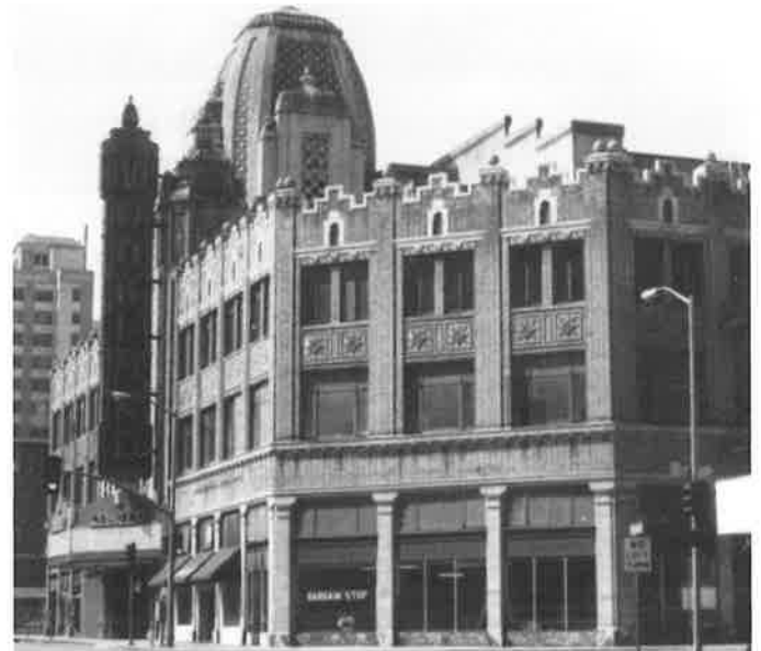
Latest reuse proposal for the Fox would revive the historic Uptown entertainment district. (Survey)
