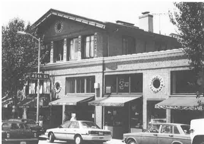
Intact period storefronts of this unique Julia Morgan commercial building will survive, thanks to vigilance and expertise of PANIL, Board, and staff. (Survey)
