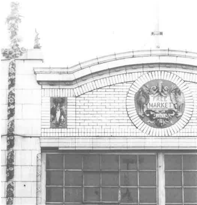
Swan's was originally built in 1917 as the Oakland Free Market. Additions over the years replicated the colorful terra cotta and white glazed brick. (Survey)
