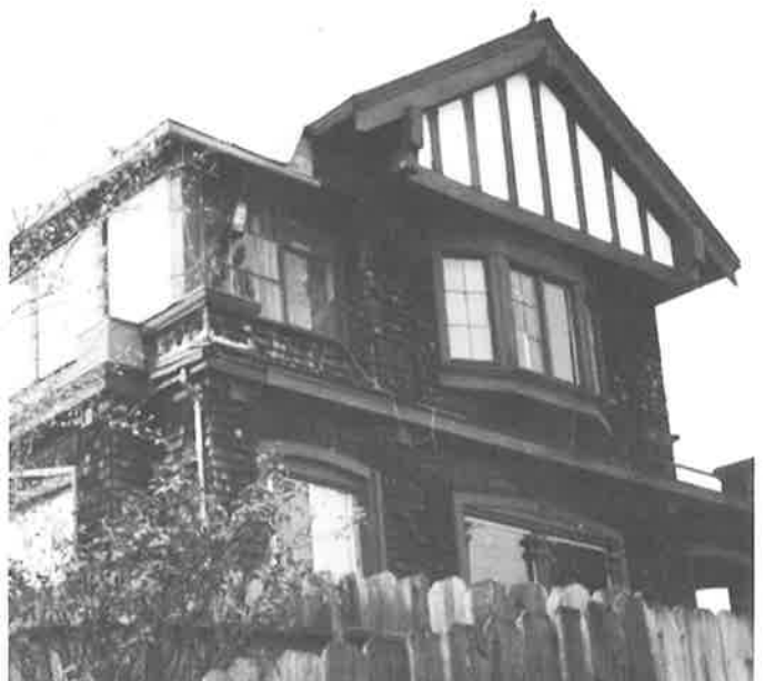
After a decade of crises and suspense, Julia Morgan's McElroy house at 401 Lee Street in Adams Point has been saved, and new owners have nominated it for landmark status: see February and March reports.
