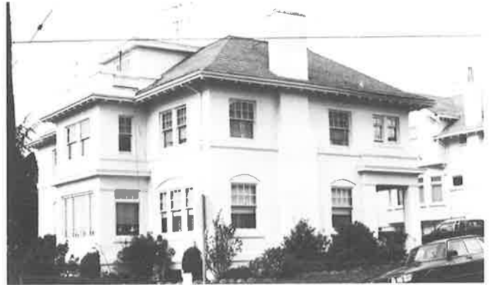
The Charles Bates house (C.W. Dickey, 1907) illustrates how Oakland's leading citizens and architects were drawn to Adams Point after 1906. (Survey)
