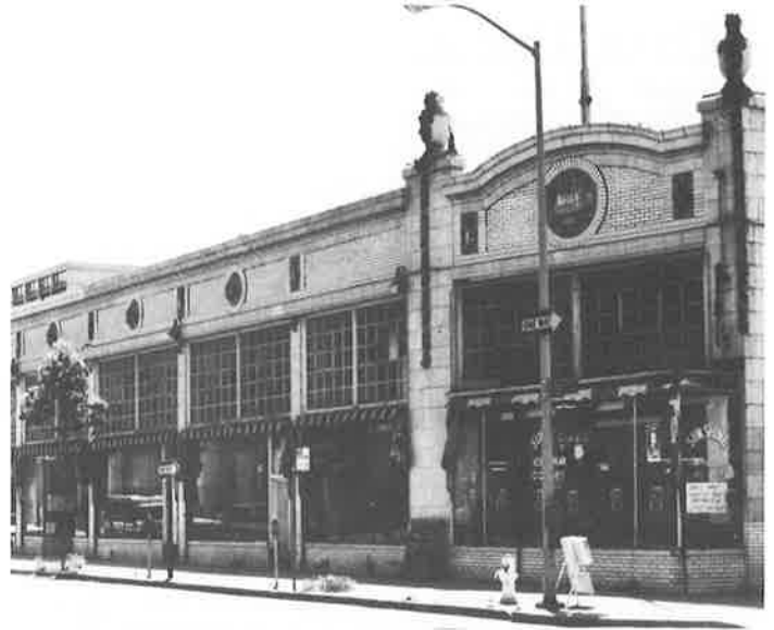
Tenth Street frontage of Swan's, before the earthquake, showing terra cotta ornament and large glass transoms and storefronts. Building is now boarded up; the plywood is adorned with Jim Kushera's swan-motif mural based on a 1950s menu from Swan's Coffee Shop in the building. (Survey photo)
