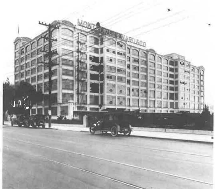
This late-1920s view of Ward's, looking southeast on East 14th Street, shows its glass and concrete construction and vigorous geometric detailing, now partly concealed by parking structure and storefront additions. (Oakland History Room)
