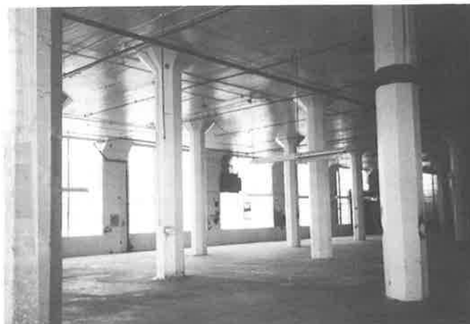
Nabisco plant, recently proposed for apartment conversion, returns to industrial use. (Betty Marvin)
