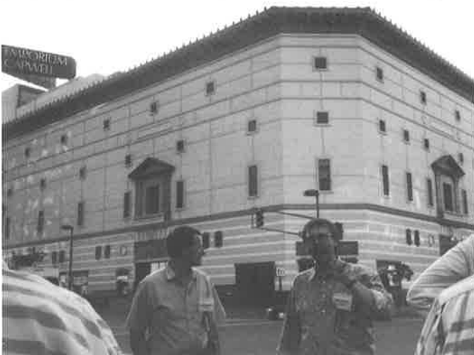
Natural disasters give preservation an element of uncertainty: Survey coordinator Gary Knecht and architect Larry Mortimer lead a National Trust tour of Oakland two years after the earthquake - the day before the hills fire. Capwell's survived the quake and reopened for business, but the brick and terra cotta Beaux Arts building was totally remodeled.
