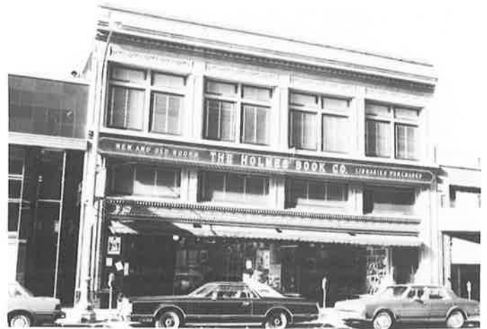
Holmes Books is an Oakland institution. Its 1925 building, with recessed storefronts and terra cotta trim, is a fine intact example of '20s commercial architecture. (Survey photo)
