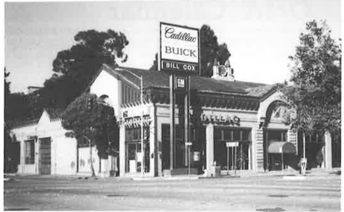
The Gothic revival Don Lee Cadillac building, redesigned by Clay Burrell in 1925 from cable car powerhouse. (Survey photo)
