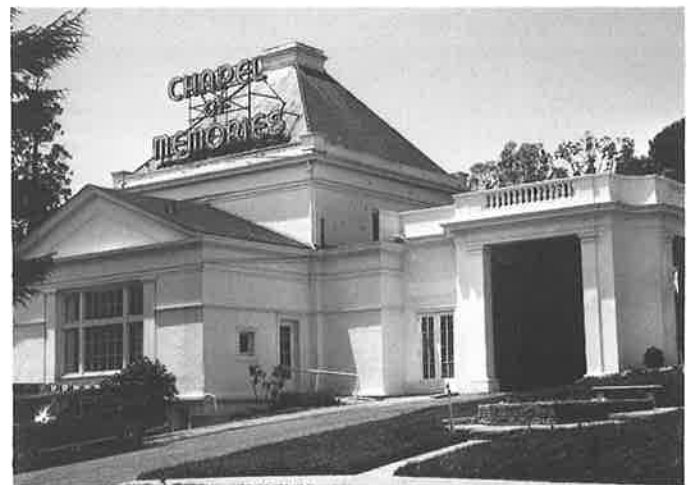
Chapel of Memories demolition aroused anger, controversy, and a closer look at demolition regulations. When this innovative crematorium was built in 1901, it was called a return to the dignified funeral practices of the ancients. (Survey photo)
