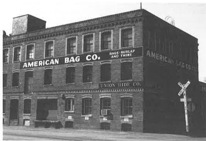
American Bag building, with its polychrome 3D brickwork, is one of the anchors of the Waterfront Warehouse District. The buildings proposed for demolition, adjoining it on the right, are less showy but supporting buildings in the district.
