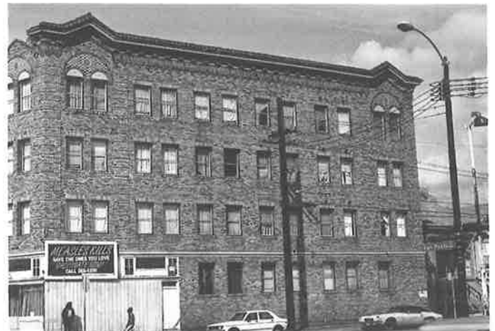
Ebony Plaza before the fire: parapets on this side survived the earthquake but are now gone. (Survey photo, 1991)
