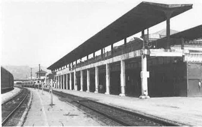
Intermodal surface transportation: S.P.'s mainline trains used the ground level tracks at the 16th Street station, while interurban tracks connected to the elevated platform. (Phil Bellman)
