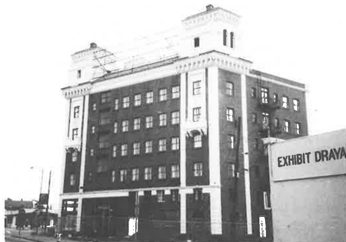
Twin towers of the California Hotel (Clay Burrell, 1930) beckoned travelers from the north (Don Hausler)
