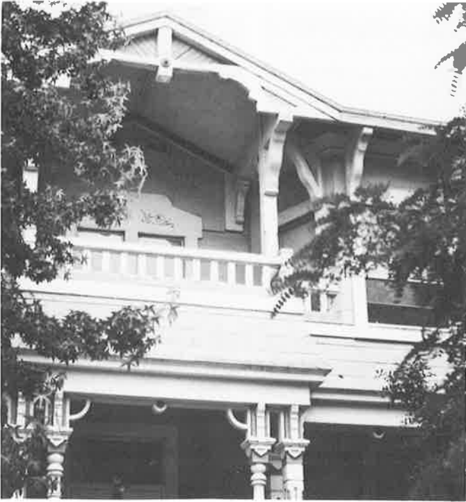
Stick details on real estate magnate John Winfield Pearson's 1884 home at 1717 Myrtle reflect the period when Oak Center development was at its peak. This style is rare elsewhere in Oakland. (Oakland Cultural Heritage Survey)
