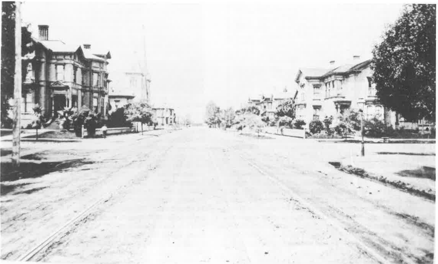
APPROACHING THE OAK CENTER NEIGHBORHOOD ALONG 14TH STREET ABOUT 1895. THIS IS THE BLOCK FROM CASTRO TO BRUSH, NOW THE FREEWAY OVERPASS, JUST WEST OF FIRST UNITARIAN CHURCH. JULIA MORGAN'S CHILDHOOD HOME WAS AT THE RIGHT, ACROSS FROM FIRST BAPTIST CHURCH. (OAKLAND HISTORY ROOM)
