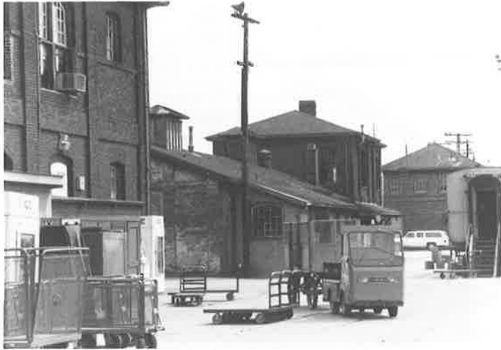
The Southern Pacific Yards and Shops historic district at the foot of Wood Street was Oakland's biggest industry in the late 19th century, building and repairing rolling stock and prefabricating buildings and bridges for most of S.P.'s
