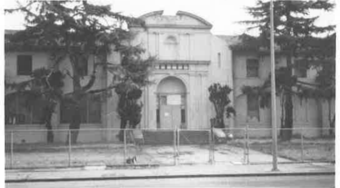
Recent tour showed a large group the damage inside boarded-up Old Merritt, as well as the quality of the interior spaces.
