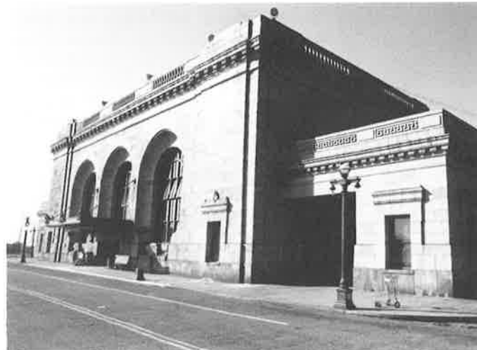
Isolated but not forgotten, the station at 16th and Wood has been the subject of City efforts to enforce repairs under the Earthquake Repair Ordinance. (Phil Bellman)
