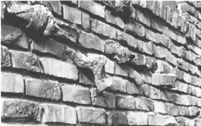
Clinker brick base distinguishes Craftsman-style Madison Park Apartments (C.M. MacGregor, 1908), to be rehabbed. (Survey)
