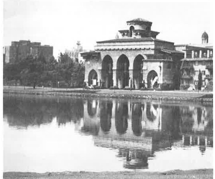
Demolition of Maybeck's Packard showroom (1929-1973) spurred landmarks legislation in Oakland. (Oakland History Room)
