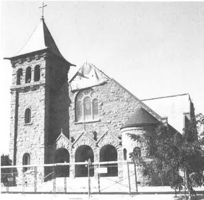
Sacred Heart Church, designed by Etienne Garin in 1901, is distinguished by Colusa sandstone walls, Romanesque-Arts and Crafts design, and monumental forms. (Phil Bellman)
