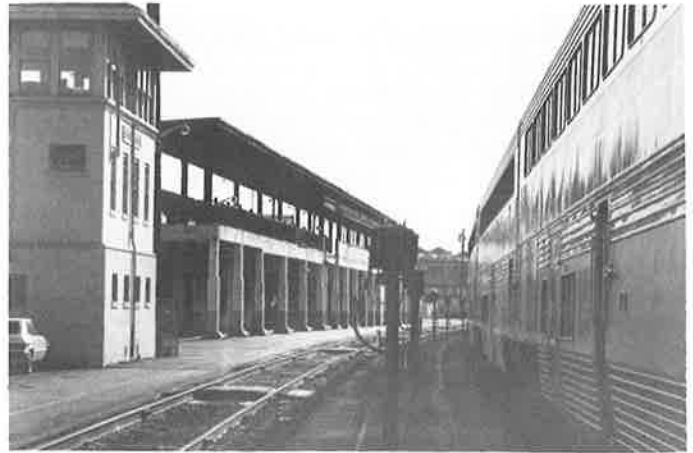
S.P. station at 16th and Wood (1910-12, Jarvis Hunt, arch.) is affected by both Cypress freeway replacement and plans for new Amtrak station at Jack London Square. (Phil Bellman)
