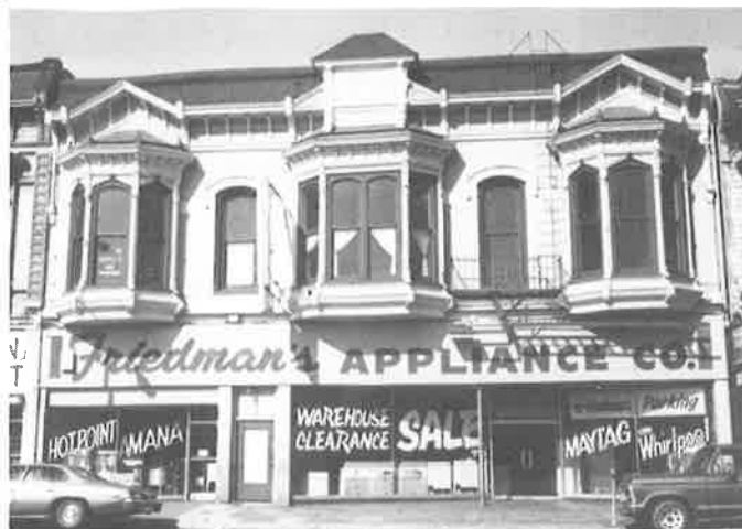
The Dalziel Block, 1878, on San Pablo near 20th Street, is a contemporary of the better-known Victorian commercial buildings of Old Oakland. (Oakland Cultural Heritage Survey, 1982)
