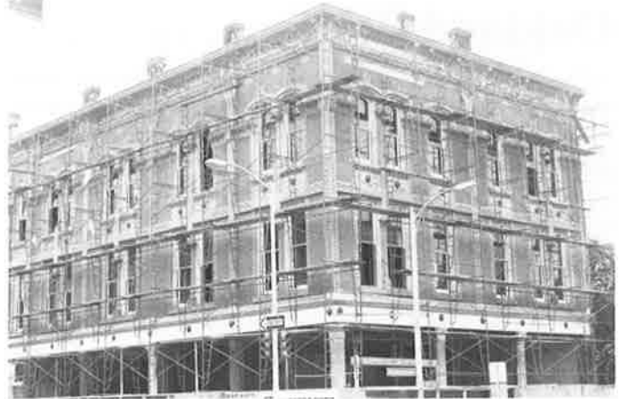
Work in progress on the LaSalle Building, 1985. Note Washington Street side with later iron columns in place of original shear wall. (Oakland Cultural Heritage Survey)
