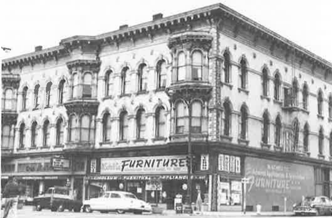
1963 photo of Ratto's building (the Gooch Block, 1876, John S. Tibbals, arch.) shows shear wall along 9th Street, and ornamental iron anchor plates. (City Planning Dept.)
