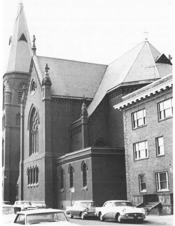
St. Francis de Sales (and rectory behind on 21st Street) in 1963, when brick was red. (Oakland Cultural Heritage Survey)
