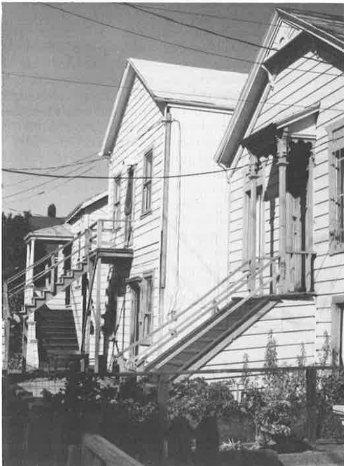
Close-set raised basement cottages in South Prescott date from early years of the transcontinental railroad. (Survey)
