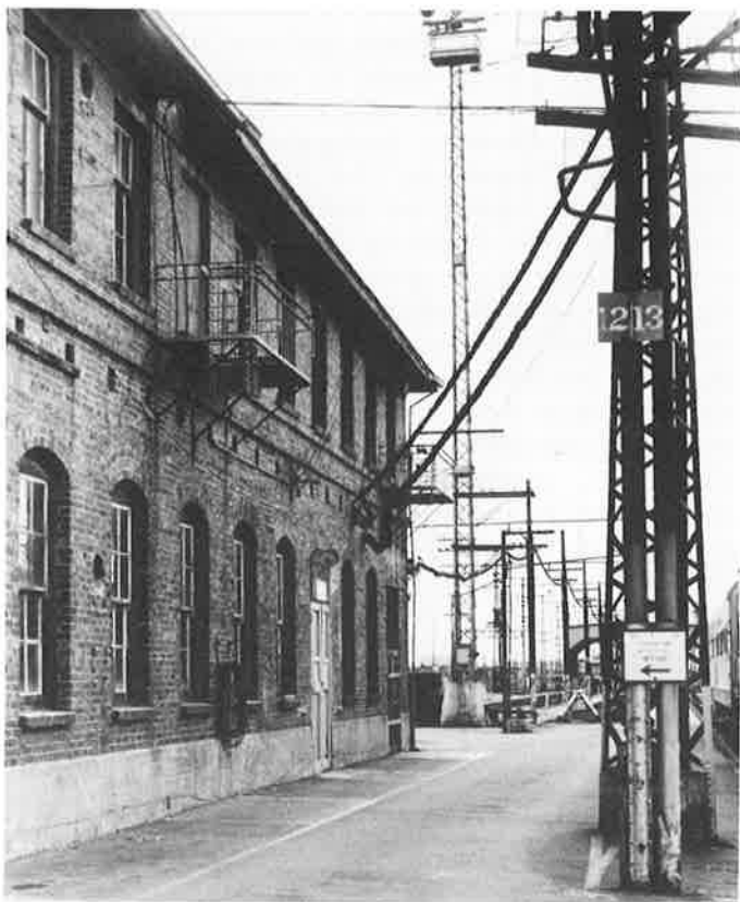
Proposed freeway route will remove all four of the early brick buildings in the S.P. West Oakland Shops District, relics of Oakland's role as the transcontinental terminus. (Phil Bellman)
