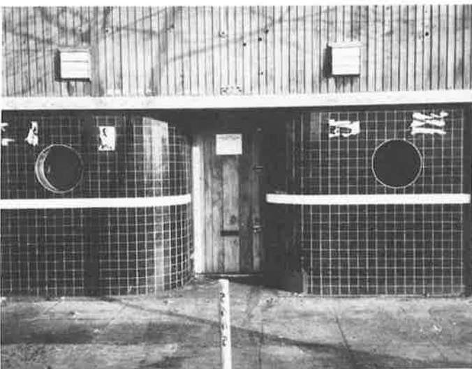
The Streamline Cocktail Lounge, 5516 San Pablo (c.1946-79), Tunnel Inn, 6041 San Pablo (opened 1930s), and Silver Slipper, 5665 San Pablo (1940-69) have typical art deco portholes, shiny tile, and stainless steel of 1930s-50s bars (Don Hausler)
