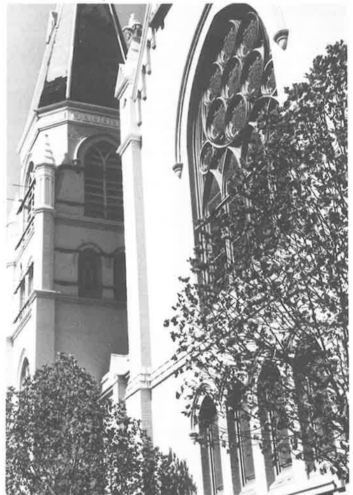
Gothic revival St. Francis de Sales (1892): Diocese feels it must be demolished, Landmarks Board disagrees. (Phil Bellman)
