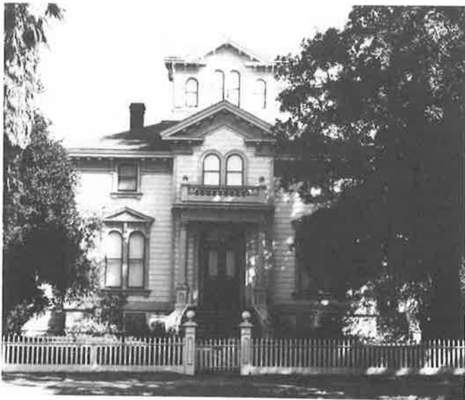
Pardee House had its brick foundation reinforced before the quake, and escaped major harm; carriage house and water tower will be repaired with FEMA aid. (Pardee Home Foundation)
