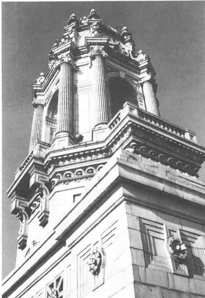
City Hall clock tower (Palmer & Hornbostel, 1911-14): rich terra cotta work shows why "replacement cost" is not an appropriate concept. (Survey photo, 1982)
