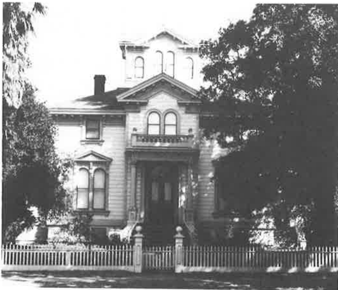
Pardee House had its brick foundation reinforced before the quake, and escaped major harm; carriage house and water tower will be repaired with FEMA aid. (Pardee Home Foundation)
