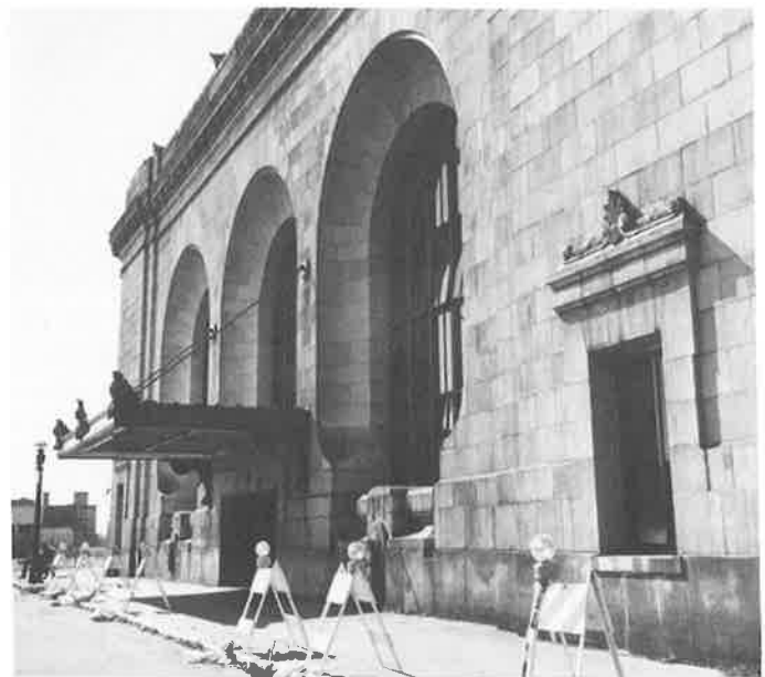
16th Street Southern Pacific Station, as a city landmark, could receive special treatment under the new earthquake repair ordinance. (Phil Bellman)
