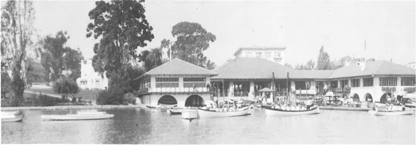
The dual-purpose boathouse and pumping station, seen from the east shortly after completion. (Oakland History Room)
