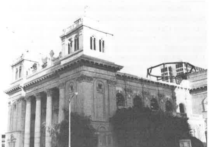
Fire remains of First United Methodist Church
